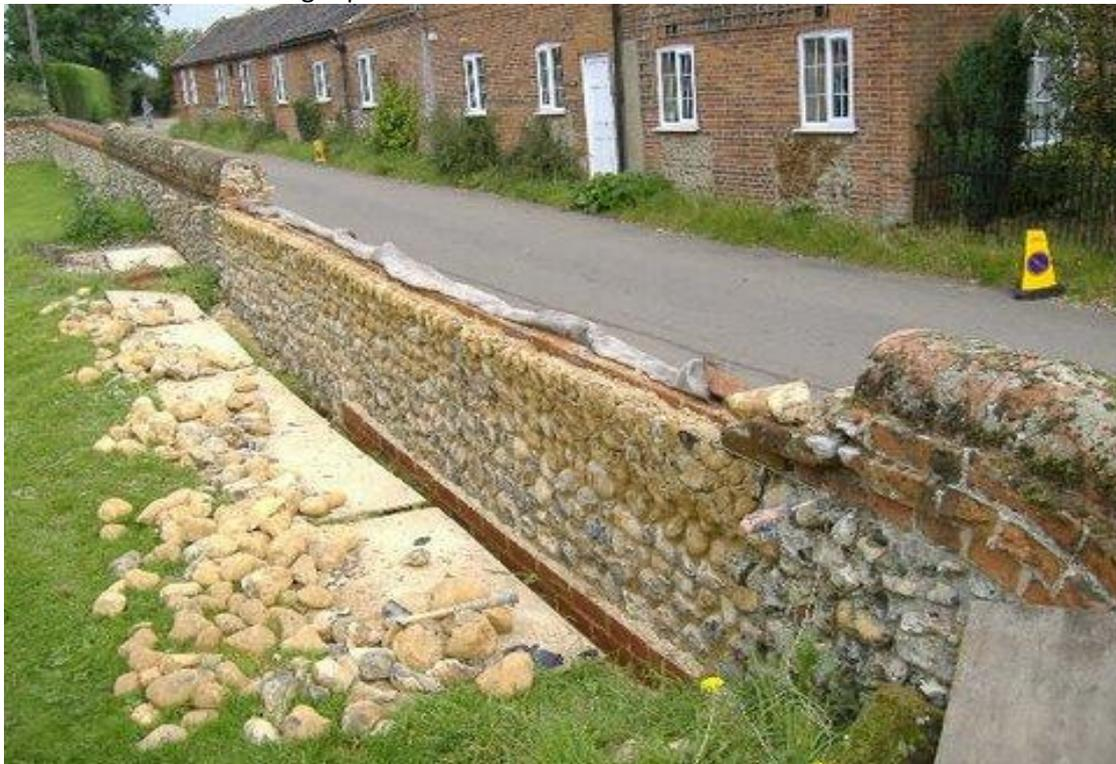
This was the worst part of the wall once the coping stones were removed from the top, the wall could simply then be pushed over
